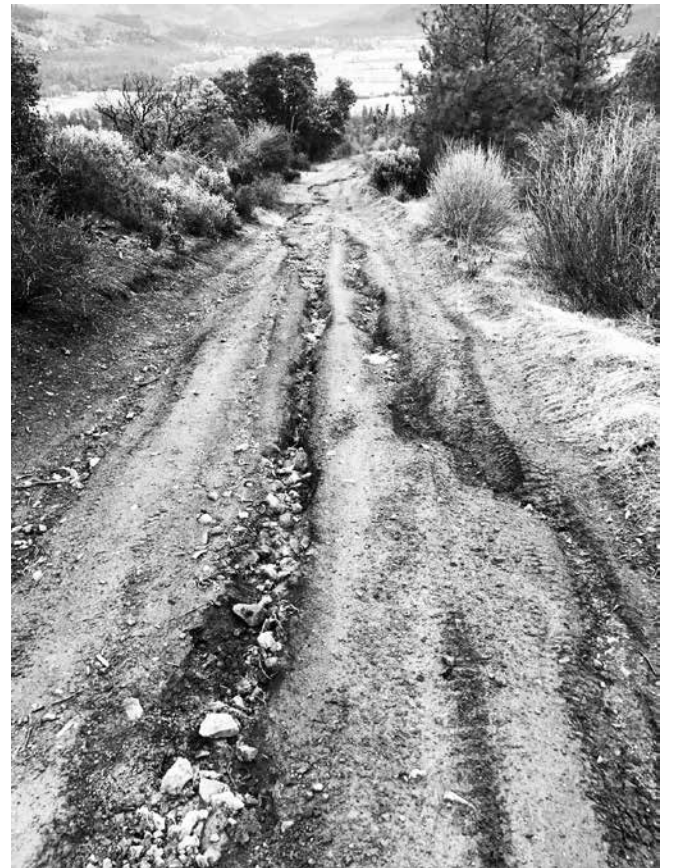
Trail ruts, some over three feet deep, have been created by OHVs on unauthorized, user-created trails.
