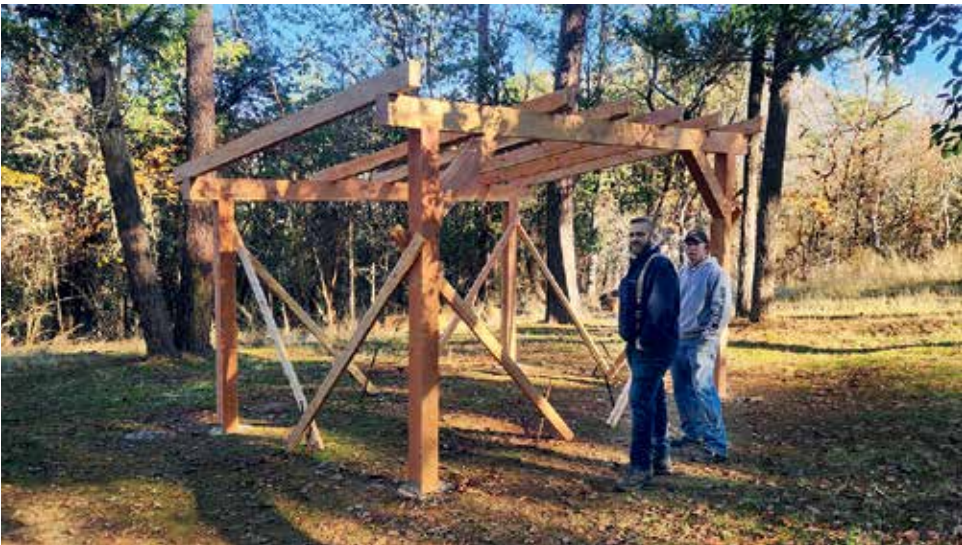
Tom Maddox (left) and Cody Goodnough working on the Hiker-Biker Shelter, which was constructed by local contractors using dead trees harvested from Cantrall Buckley and milled locally by 4M Timber. Photo: APWC.
