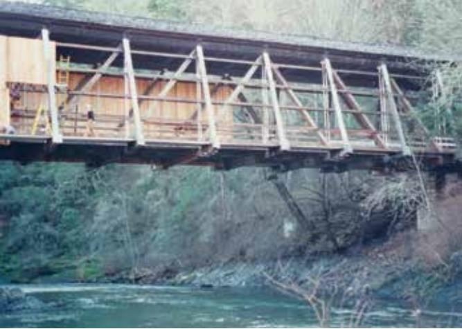
New siding on McKee Bridge in 1995.
