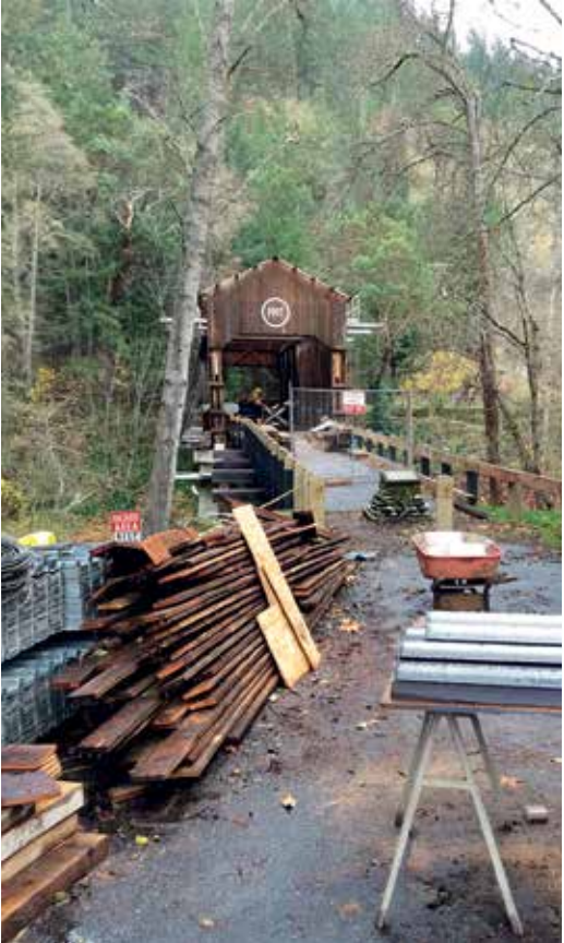
McKee Bridge under renovation.
