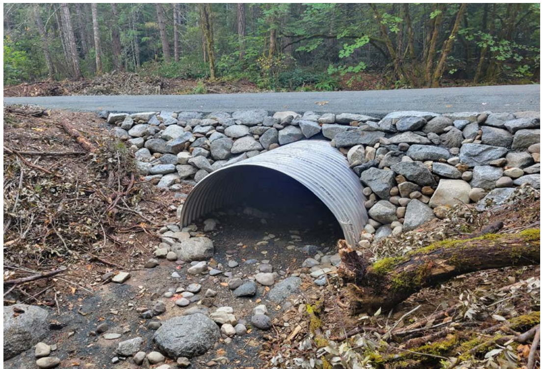
After: New embedded culvert with a natural streambed, allowing fish and water to move freely. Photo by Luke Wimmer, Applegate Partnership.
