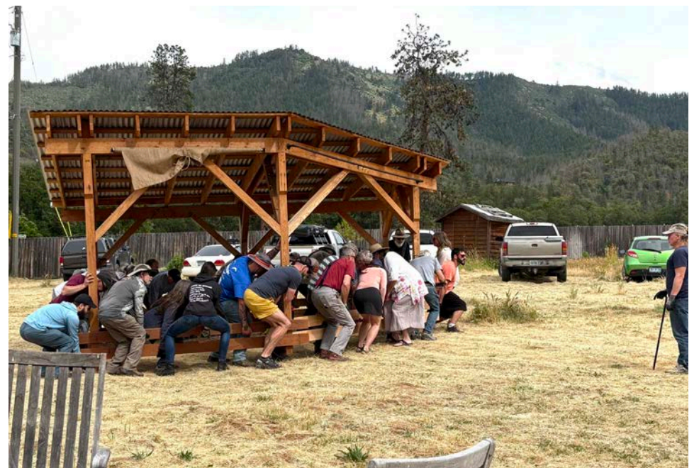
Community members join forces to move a shelter by hand during a barn-raising-style event in the Applegate Valley. Photo by Christina Ammon.
