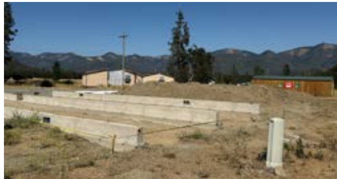
Construction for Pacifica classroom space, makerspace, and nature center. Photo by Vanessa Redding.
