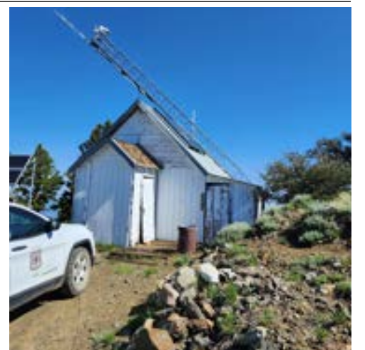
The Dutchman Lookout ground house had been neglected for many years and suffered significant damage when heavy snow in the winter of 2022 caused the communication tower to collapse onto the roof. Photo by USDA Forest Service, Michael Ingman.
