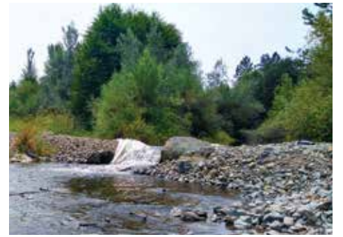
Even though the dam is only three feet high, it can trap juvenile fish. Photos: APWC.
