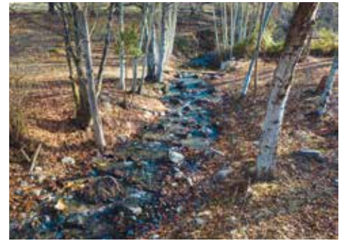
A reconstructed roughened channel near Talent that’s similar to what’s planned for Williams Creek.
